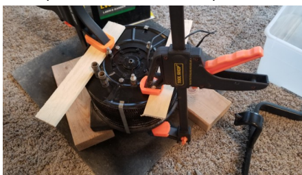
Clamped for Removal or Replacement
